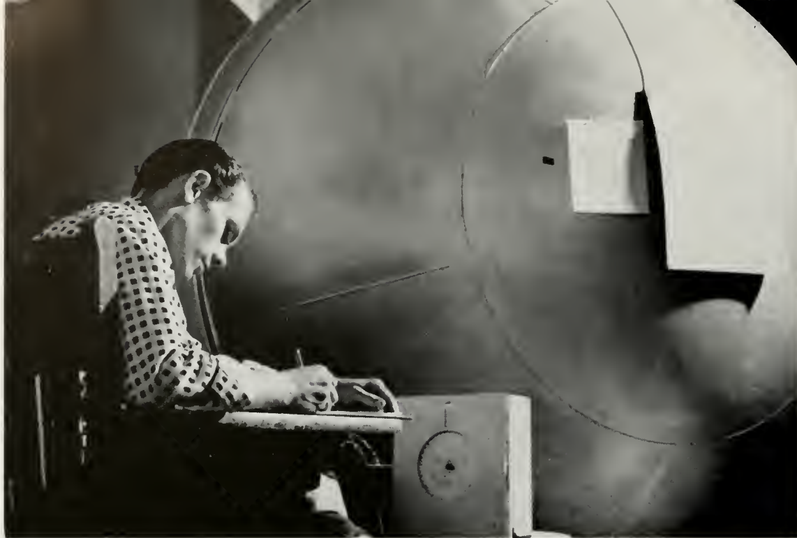
Eight feet in diameter, this integration sphere was large enough to hold a man. It was painted white inside for the purpose of investigating the effect of the visual environment on behavior. Incandescent, sodium and mercury lamps were used for studying types of illumination and visual fatigue.
